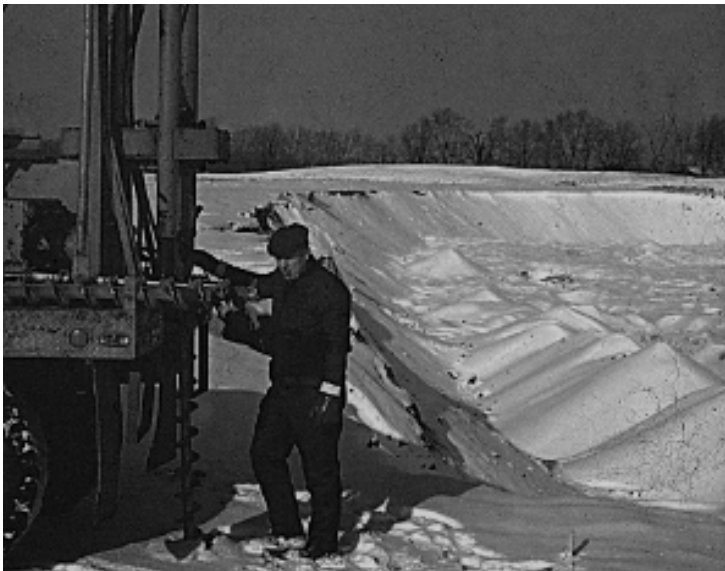
Soil sampling with the Mobile B-52 in 1968
